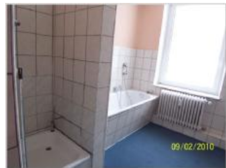
Bad - Haus links - 1.OG
